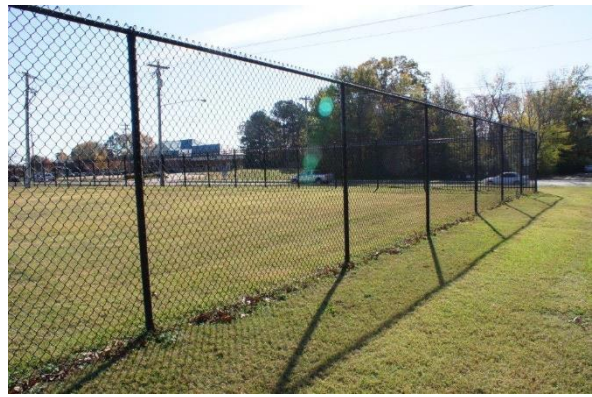
Figure 3 Chain Link Fencing Example
